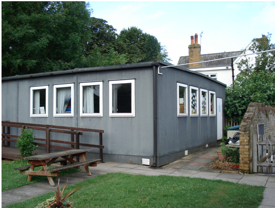
View looking west along proposed classroom block site towards 21 School Lane
